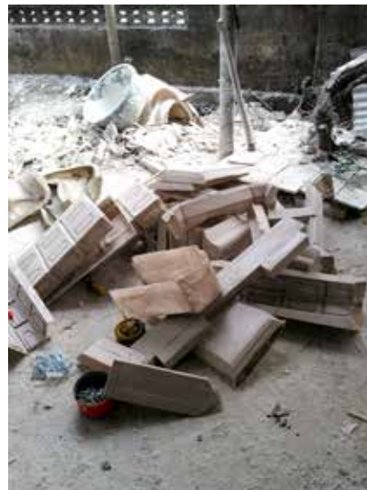
Monuments, 2017 In progress / Moulds Photo: Kotot
